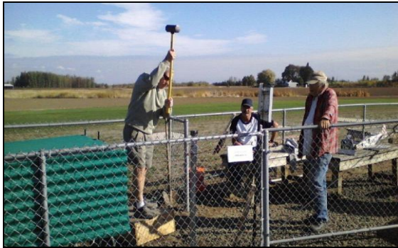
Second well down 15 feet. Flow not good yet, but working on it.
