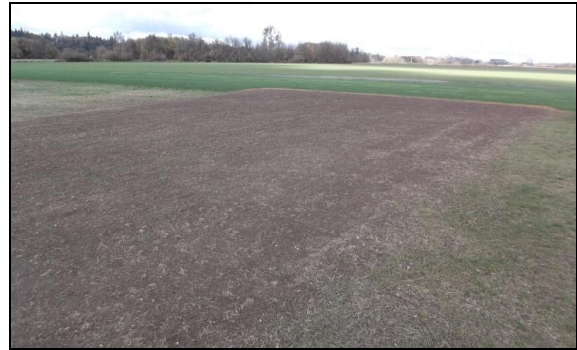
Geotex runway area rototilled, dragged and Roundup applied.
