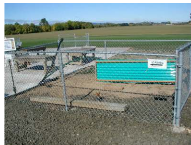
Pump stored for winter
