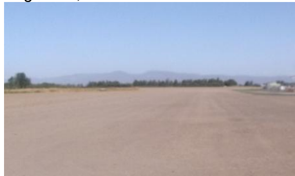
Leveled and rolled
